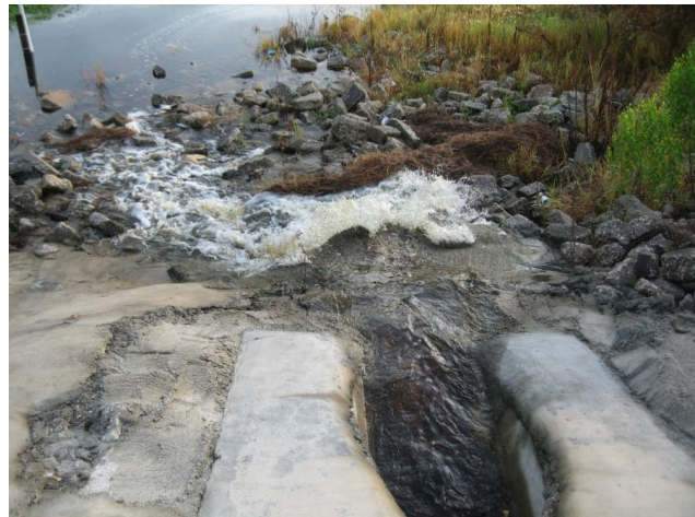
c. Discharges from 30-inch RCP During Storm Conditions
