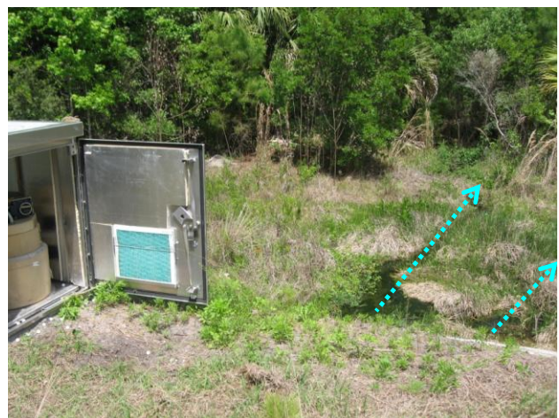
b. Flow Discharges into Wetland Treatment Area
