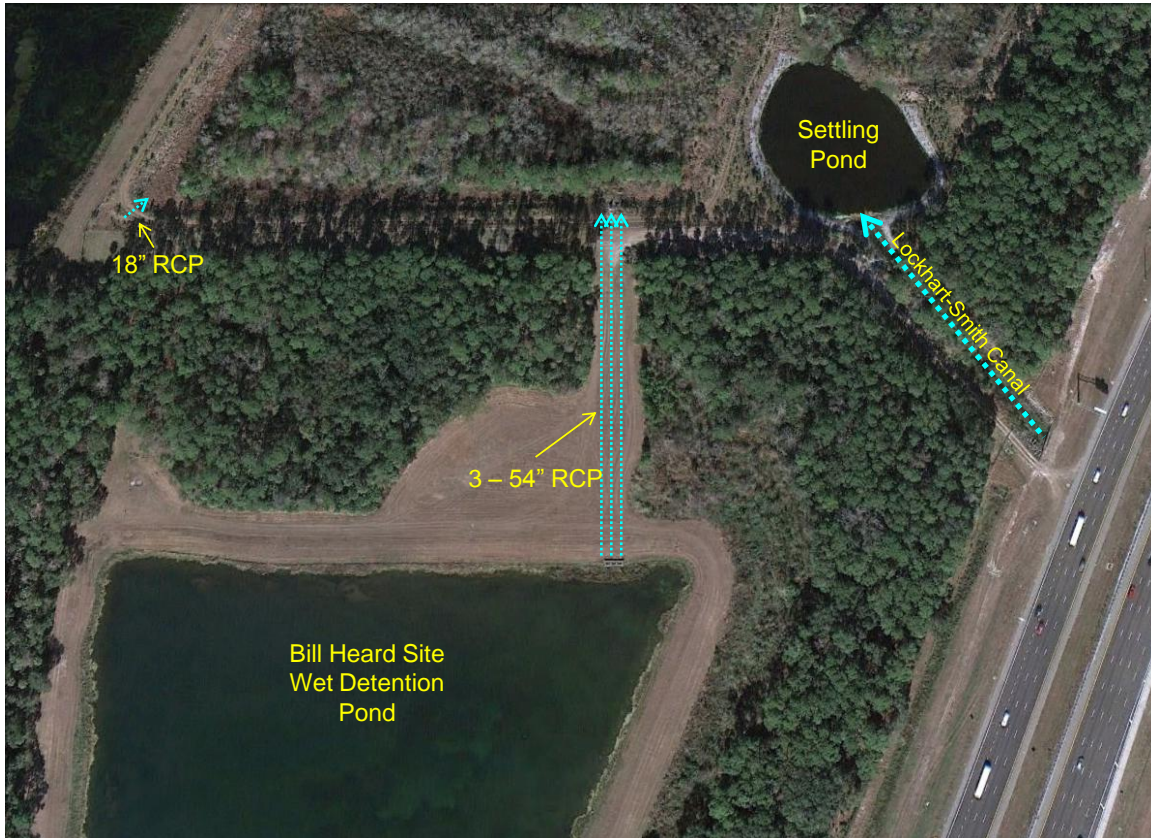
Figure 1-6. Hydrologic Inflows in the Southern Portion of the Lockhart-Smith RSF.
